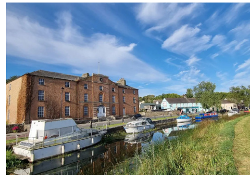
6. Former Grand Canal Hotel
