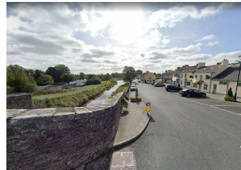
3. View from Binn's Bridge (south)
