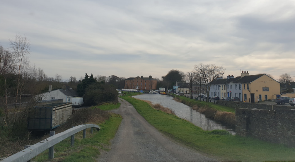
View from Binn's Bridge
